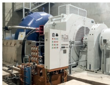
Sap Viet, Vietnam 23.5 MW; two large horizontal Francis units in South-East Asia
