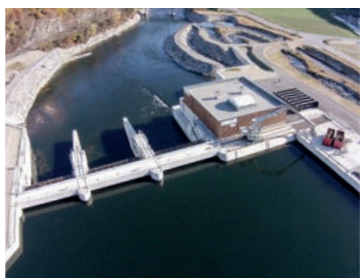
Rothleiten, Austria 5.10 MW; important Bulb turbine reference in Europe
