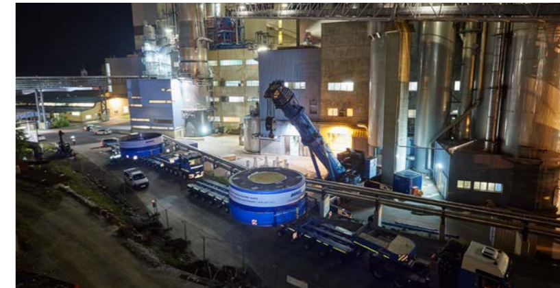
The giant steel Yankees are delivered in two halves and assembled on the customer's site.
