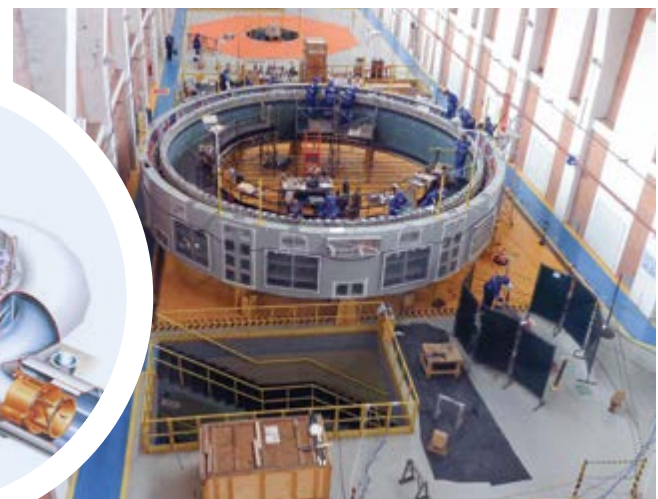
The generators for Belo Monte have a generation power of 679 MVA and impressive internal diameter of the stator of 18.5 m.
