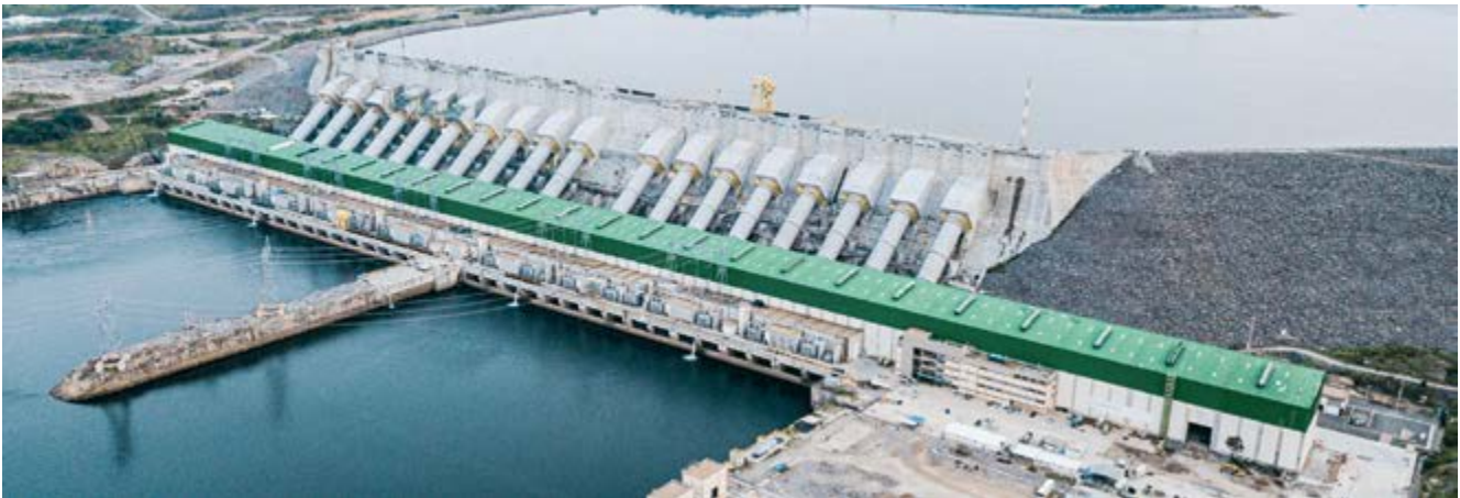
The main powerhouse Belo Monte houses 18 vertical Francis units with a total capacity of 11,000 MW, making it the world's third largest hydropower plant.
