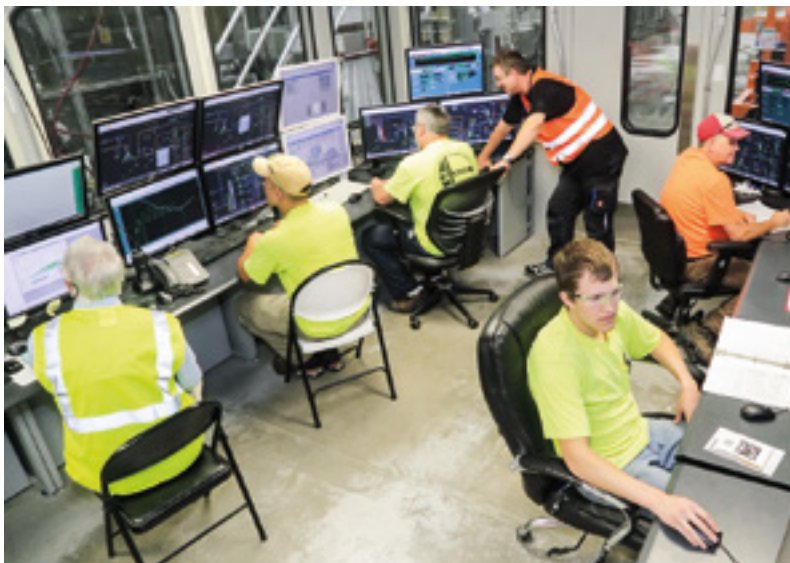
▲ Operators in the control room for TM1 and TM2.
