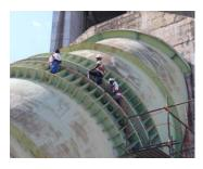
Inga II, DR Congo 2013; 1,424 MW Complete renewal of penstocks, intake trashracks and gate rehabilitation Head / Length: 93 m / 110 m Diameter: 8.0 - 6.5 m Total weight: 2,745 tons
