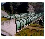
Mingtan, Taiwan 1989; 1,602 MW Penstocks and conduits Head / Length: 575 m / 2,000 m Diameter: 7.5 - 2.3 m Total weight: 25,949 tons
