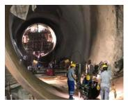
Yusufeli, Turkey 2016; 558 MW Penstock, gates, trashracks, spillway, hydraulic lifting systems, and valves Head / Length: 255 m / 245 m Diameter: 9 - 3.8 m Total weight: 5,350 tons
