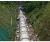
Pirris, Costa Rica 2010; 138 MW Exposed penstock and steel liner, bifurcator and spherical guard valve
