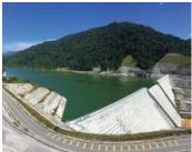
Ulu Jelai, Malaysia 2013; 382 MW Penstock, manifold, high head gates, stop logs, trashracks, desilting system Head / Length: 359 m /200 m Diameter: 5.2 - 2.5 m Total weight 1,133 tons
