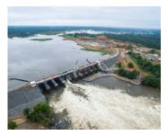
Mount Coffee, Liberia 2014; 64 MW Rehabilitation of hydromechanical equipment for the second largest HPP in Liberia Head / Length: 35 m / 45 m Diameter: 5.3 m Total weight 900 tons
