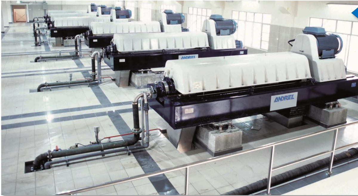
ANDRITZ decanter centrifuges for Sungai Semenyith, Malaysia, one of the largest drinking water treatment plants in South East Asia
