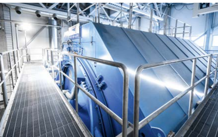
The delivery also included a new DD-Washer for brown stock washing, new screening plant, and new refiners.
