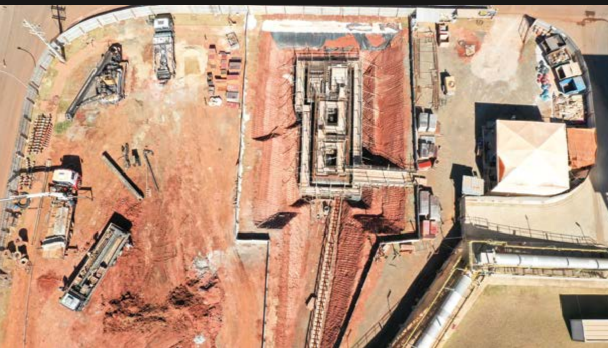
Status of the on-site construction works in May.
