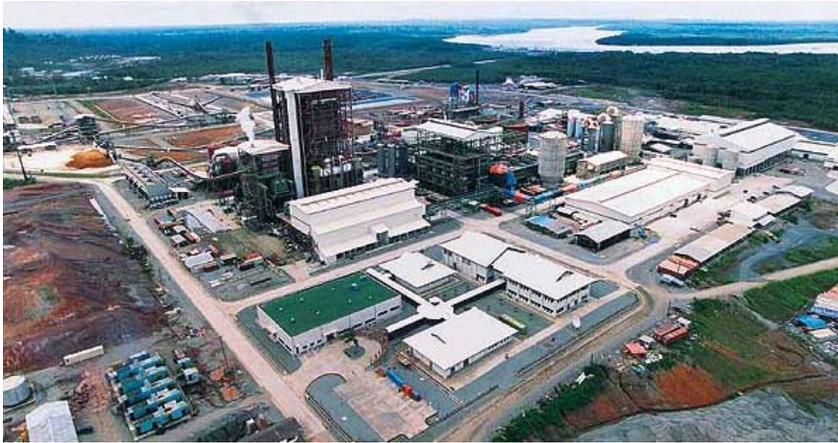
P.T. Kiani Kertas has built a bleached kraft hardwood pulp mill in East Kalimantan, Indonesia. The mill is designed to produce pulp at a capacity of 1500 ADMtpd (air dry metric tonnes per day) initially from mixed Indonesian hardwoods and eventually from plantation Acacia and Eucalyptus. The mill incorporates state-of-the-art technology which satisfies both environmental and process demands.
