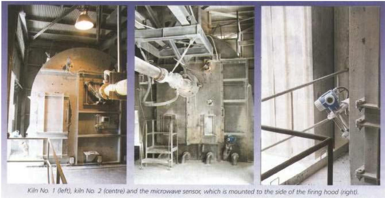
*Kiln No. 1 (left), kiln No. 2 (centre) and the microwave sensor, which is mounted to the side of the firing hood (right).*
