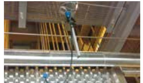
▲ ACU sensors installed on recovery boiler
