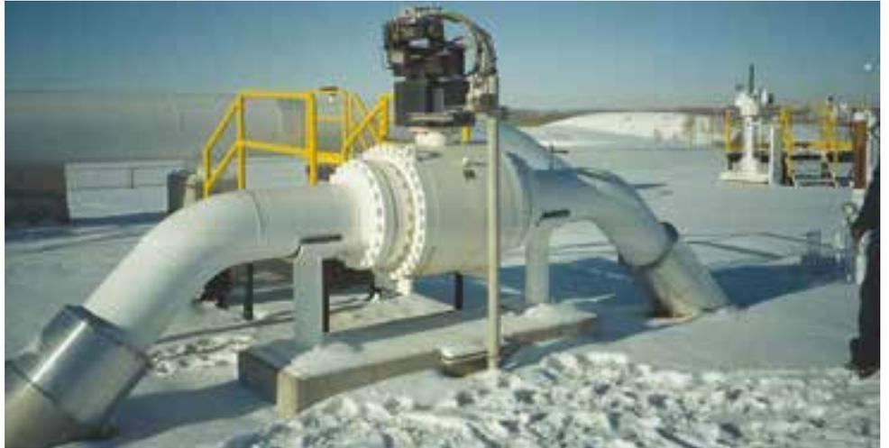
A challenge on the line involved the replacement of a 25-year-old control valve installation that Enbridge operators had found extremely unresponsive. An IDEAS simulation model of the pipeline showed the existing control valve installation to be greatly oversized for the current service conditions. Several candidate replacement valves were evaluated from competitive vendor bids, including alternatives for adjacent piping geometry.
