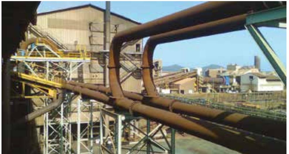
This provided considerable cost savings for the smelter, but the customer wanted the design checked thoroughly because it was so different from its existing off-gas systems. The temperature loss was critical to the success of the design because the gas needed to be down to a certain level at the inlet of the baghouse to protect the bags.
