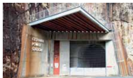
▲ Entrance to the power station tunnel at HPP Cethana
