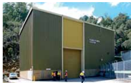
▲ Hydropower station Fisher
