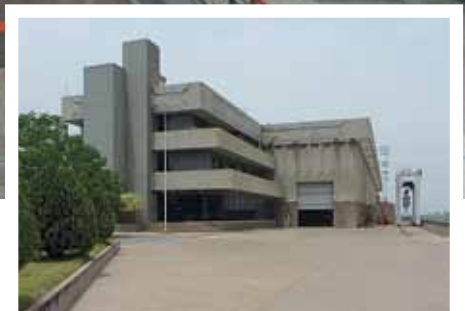
▲ Kpong hydropower plant
