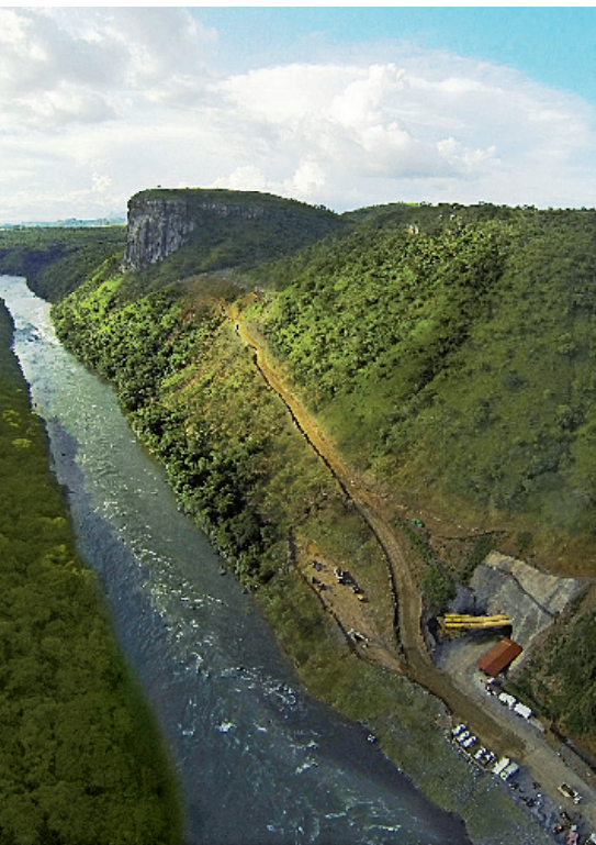
• Kwanza River and future power house access of HPP Laúca
