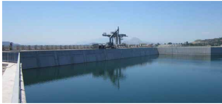
Figure2:Upstream View of Ashta 1
