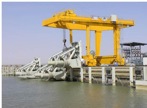
Picture 2: TG-units of Jebel Aulia Dam HM Plant in raised position
