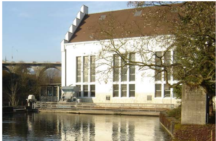
Picture 6: Existing powerhouse
