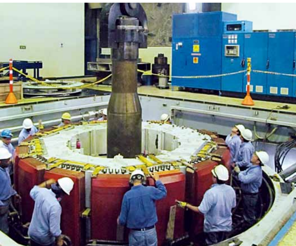
▼ Rotor installation
