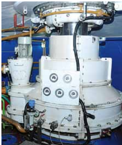
▲ Turbine pit after renovation
