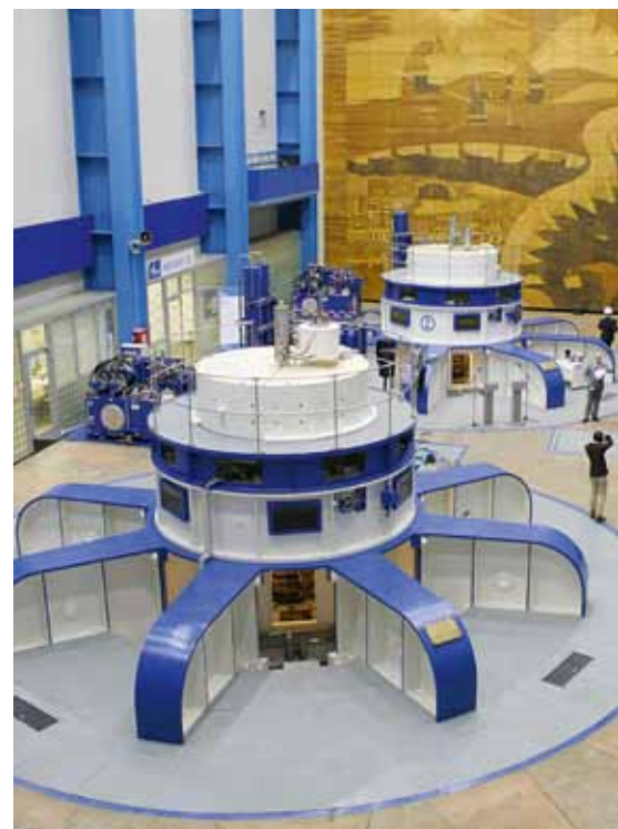
▲ Unit #1 and unit #2 after modernization
