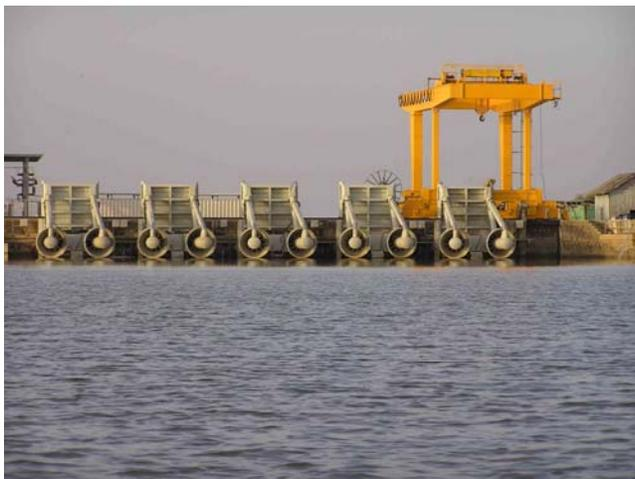
Fig. 1 – Modules at Jebel Aulia Dam housing 2 TG-Units in horizontal configuration. Modules shown in raised position from upstream side, yellow gantry crane to lift Modules, 40 Modules, total plant output 30 MW.
