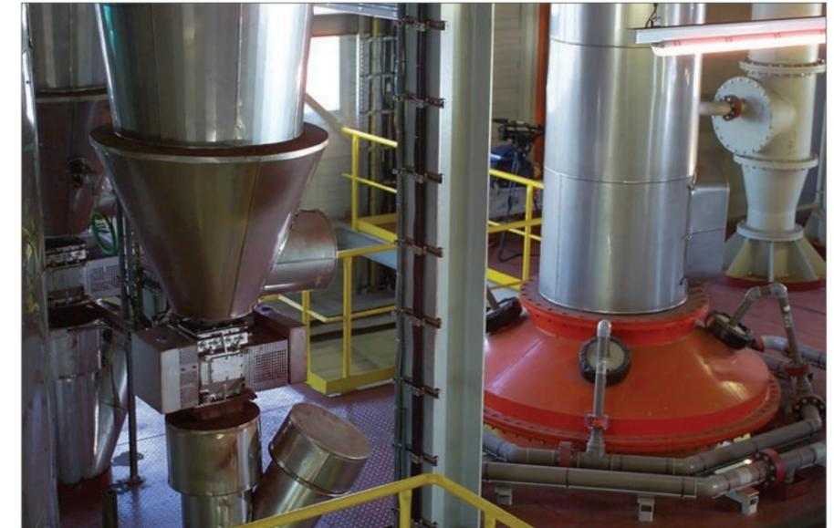
▲ Dust separator and injection of waste pickle at the evaporator
