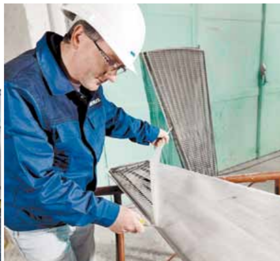
Disassembly of old disc filter segments. Removal of old filter bag.
