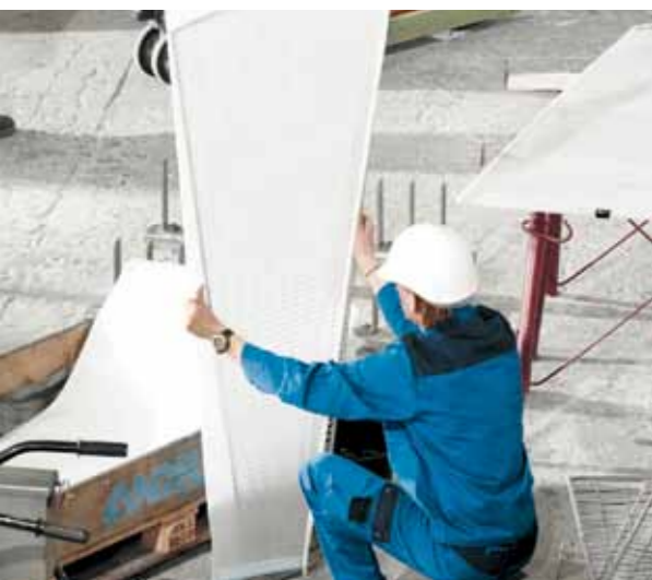
Installing new filter bag
