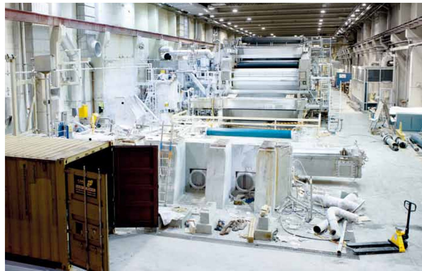
▲ A view of the machine room at UPM Kymi's mill where the machine is being dismantled and inspected. ▼
