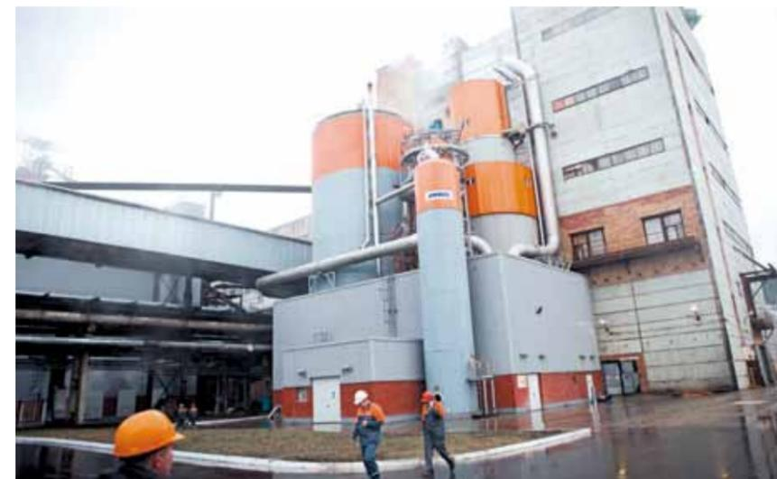
◀◀ The brownstock washing system includes new pressure diffuser (left) and new two-stage DD Washer (below).
