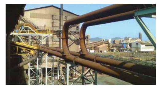
This provided considerable cost savings for the smelter, but the customer wanted the design checked thoroughly because it was so different from its existing off-gas systems. The temperature loss was critical to the success of the design because the gas needed to be down to a certain level at the inlet of the baghouse to protect the bags.
