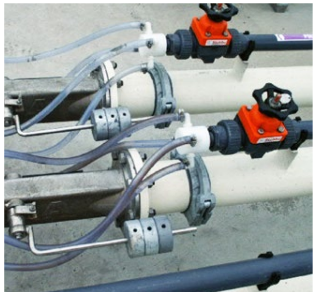
Venturi mixer, inline flocculation system
