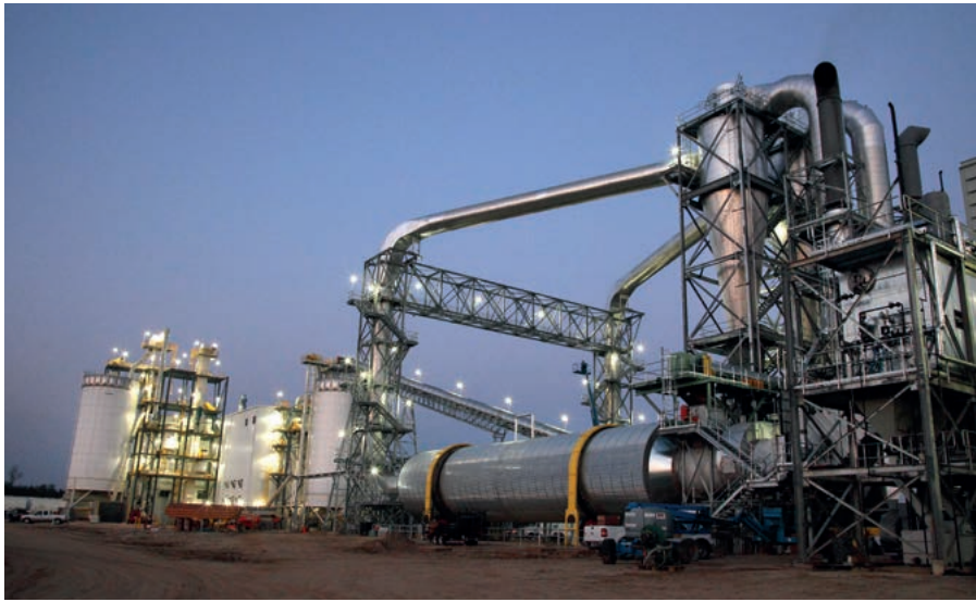
▲ It was only 14 months from the first turn of a shovel to production of the first pellet. This view shows the thermal driers and power boiler in the foreground (right) and the pellet plant in the background.
