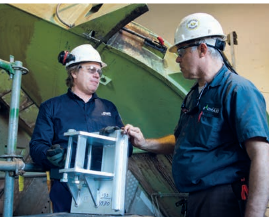
▲Timo Lintunen, ANDRITZ Service Engineer (left), reviews maintenance procedures for the chipper with Frankie Gamage, Woodyard Operator of Georgia Biomass. ANDRITZ has a maintenance service agreement with the plant for woodyard services and replacement parts.
