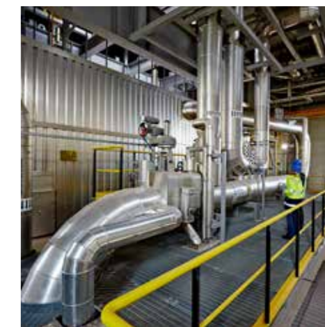
▲ The boiler's design is based on ANDRITZ's well-proven Bubbling Fluidized Bed (BFB) technology combining high fuel efficiency with excellent environmental performance.
