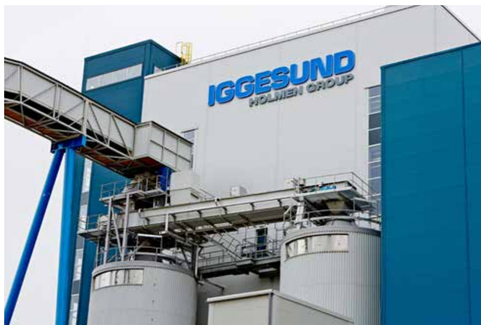
▲ Biomass feeding system to the BFB boiler
