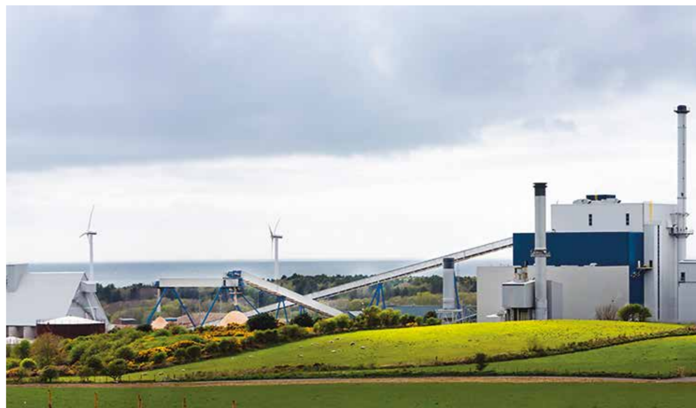
▲ New biomass boiler island for Iggesund Paperboard is located in Workington in Cumbria, United Kingdom. Photograph courtesy of Holmen Group.
