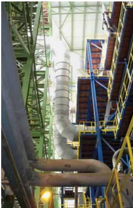
▲ Cooling air ducts of After Pot Cooling (APC) tower
