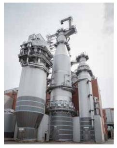
Metsä Fibre's Joutseno mill modified its fiberline to use ANDRITZ's polysulfide cooking process. This is the world's largest single polysulfide cooking plant.
