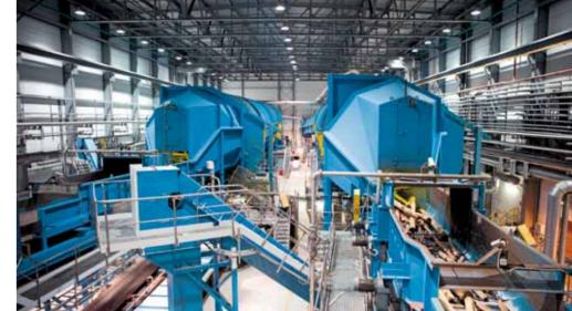
◆ The brownstock washing system includes new pressure diffuser (left) and new two-stage DD Washer (below).
