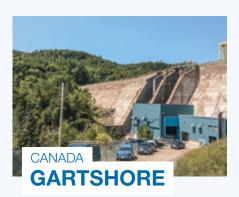
New contract; June 2017; 23.5 MW; Great Lakes Power Limited; general major rehabilitation incl. new Kaplan runner, stator winding and turbine governor; completion planned October 2018;
