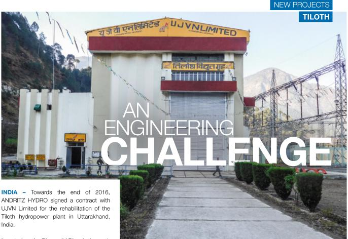
Located on the Bhagrathi River in the north of India, HPP Tiloth was originally commissioned in 1984. It consists of three generating units with a capacity of 30 MW each.
