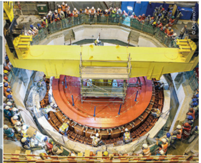
Lowering of rotor unit #1
