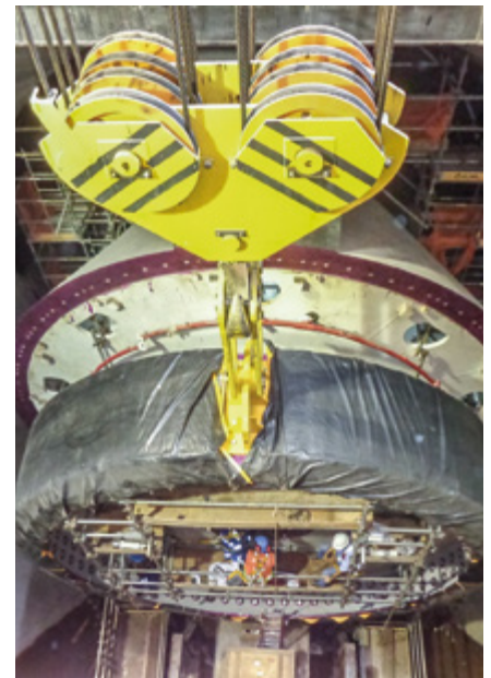
Installation of Bulb generator
