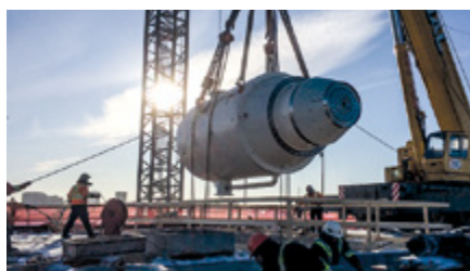
Installation of Bulb turbine
