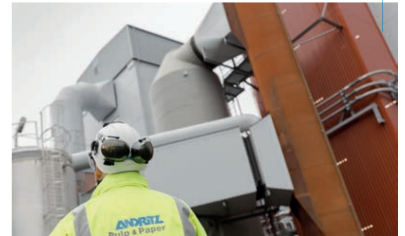
The ANDRITZ flue gas cleaning system consists of ESP, a TurboSorp system (semi-dry flue gas cleaning system), a bagfilter, and flue gas condensation. The TurboSorp plant separates the acidic components from the flue gas.
