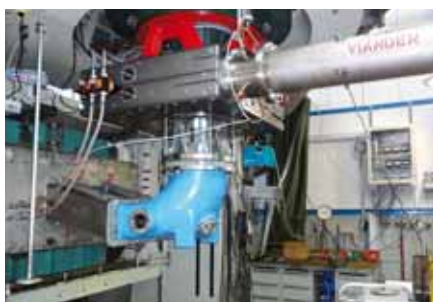
▲ Model of the pump turbine Vianden M11 on the test rig
