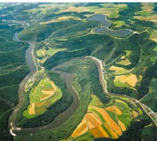
▼ Aerial view of upper reservoir of Vianden in Luxembourg
