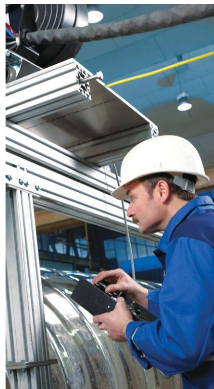
Adjusting the welding equipment
