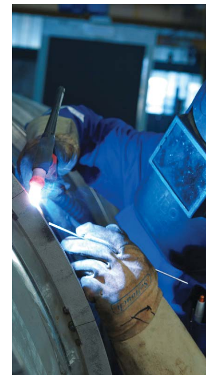
Selective manual welding of wear shoes
