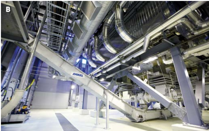
A The fuel-to-boiler connection
