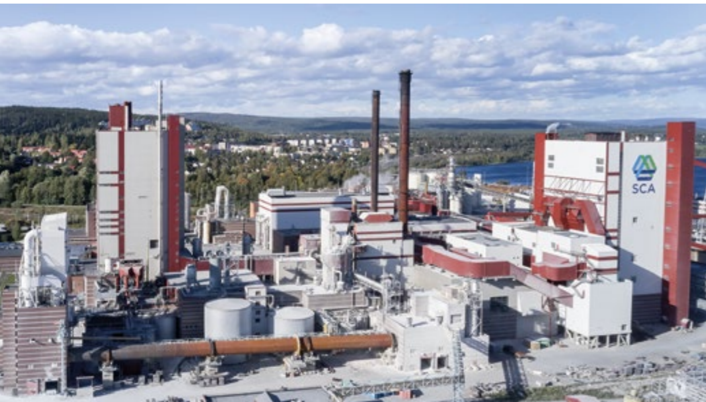
There were five start-ups in the white liquor plant during project Helios
