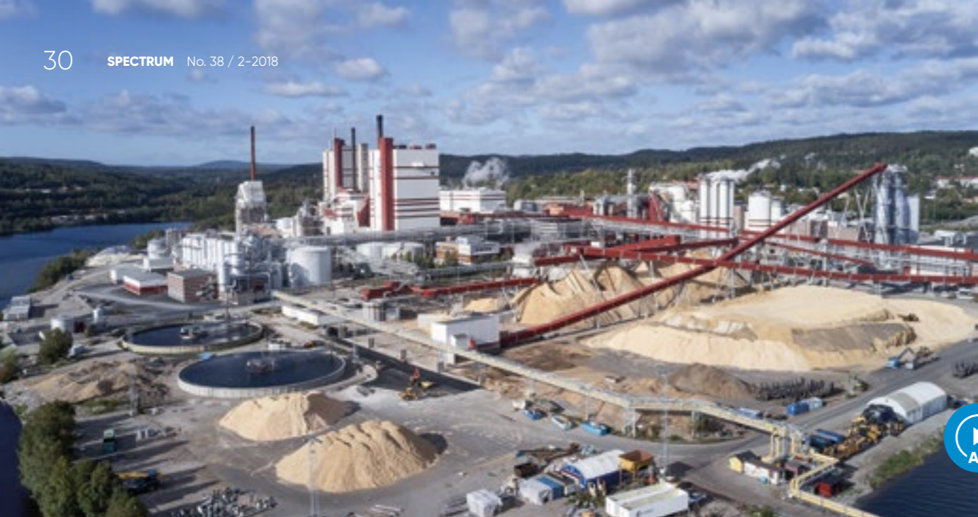
Helios project was a really well-planned and designed project in order to double the capacity, though keeping the existing mill running almost the whole time
