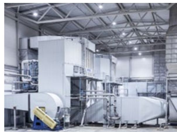
Parts of the heat recovery system located in pulp drying
