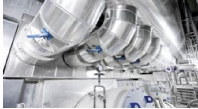
New secondary air layer for advanced air staging to reduce NOx emissions.
