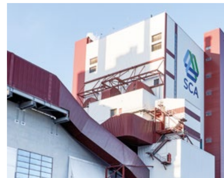
The recovery boiler was expanded by 3.8m and the capacity was increased from 3,300 to 5,000 tds/d
