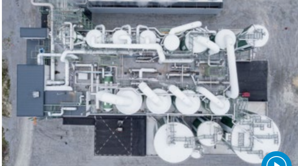
The new 7-effect high dry solids evaporation plant replaces existing evaporation lines and significantly enhances energy efficiency at the Mörrum mill
