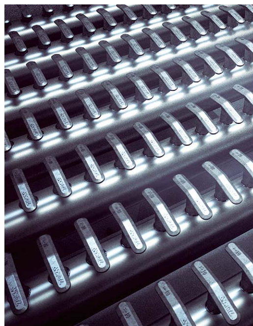
Retrofit BFB nozzle grid for waste fuel.
