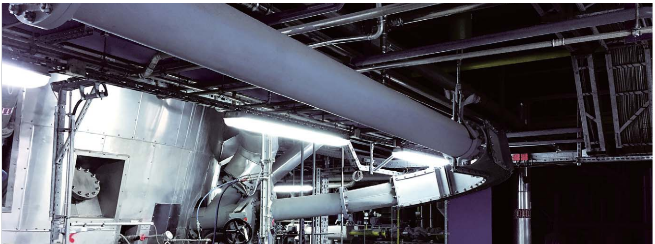
Pneumatic fuel feeding system
