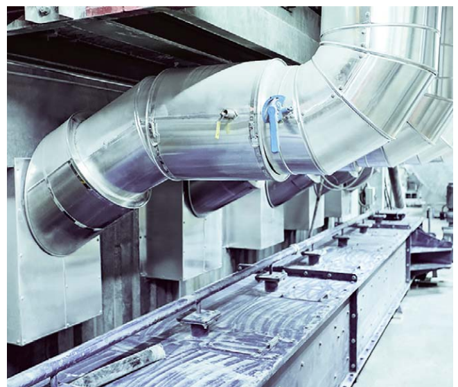
Advanced air staging and FGR upgrade
