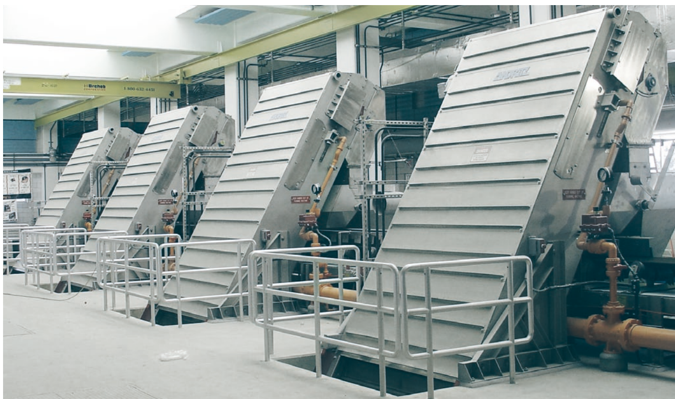
Aqua-Screen commonly used for pre-treatment
