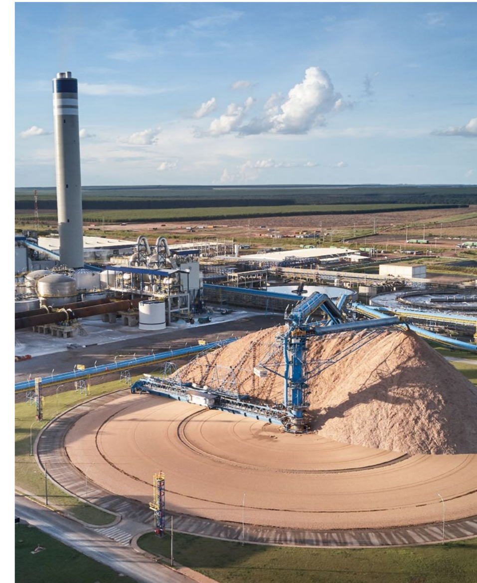
ANDRITZ delivered a complete wood processing plant with four chipping lines, each consisting of the world's biggest horizontally fed HHQ-Chippers.
