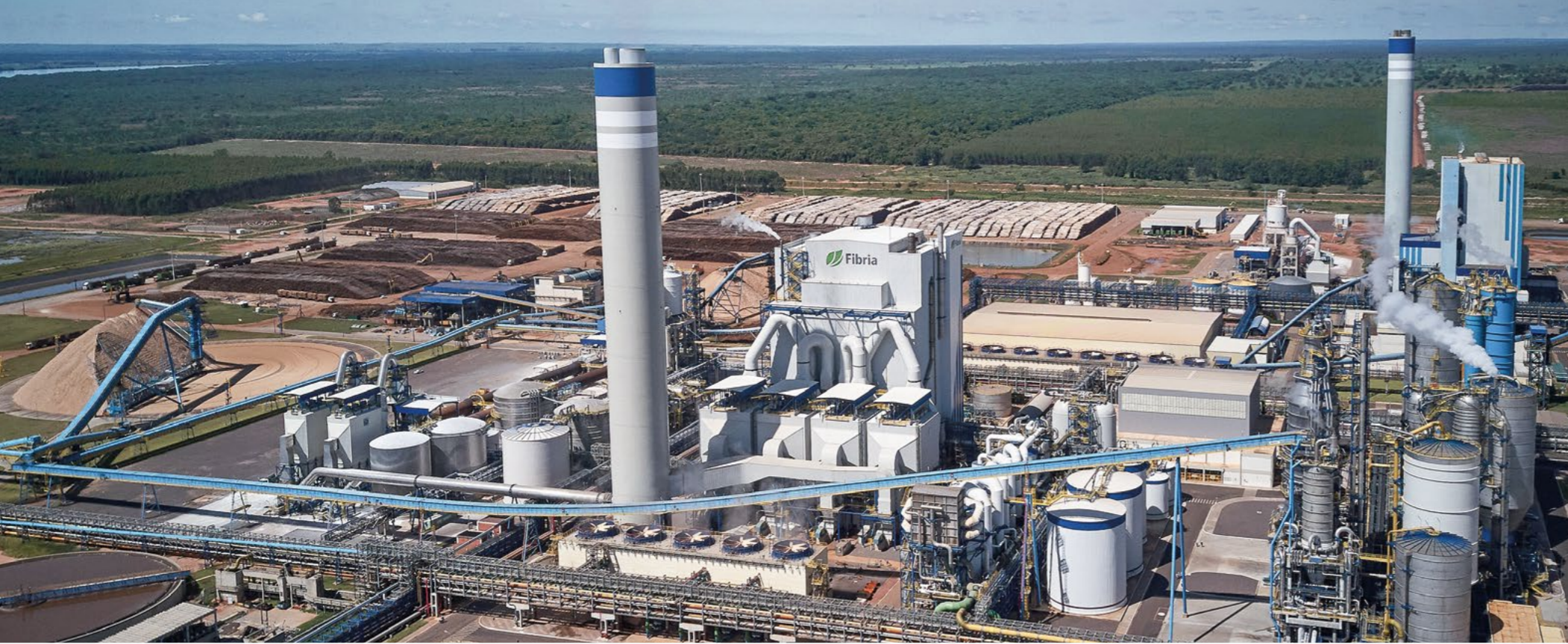
ANDRITZ teamed up with Fibria to build Horizonte 2 Project – the world's largest pulp mill with a single fiberline. The ANDRITZ scope in this full turnkey project included everything from the woodyard to the drying machines and the whole recovery island.
