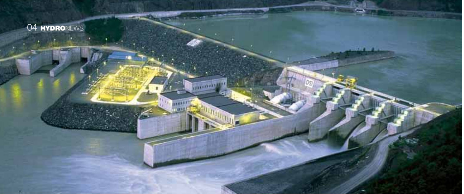
Nightview of hydroelectric power plant Muratli, Turkey
