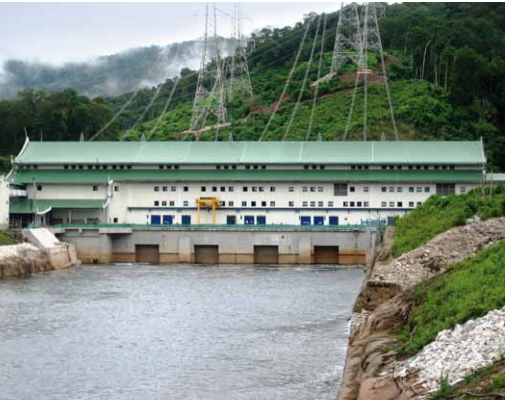
Nam Theun power plant from tailwaterside
