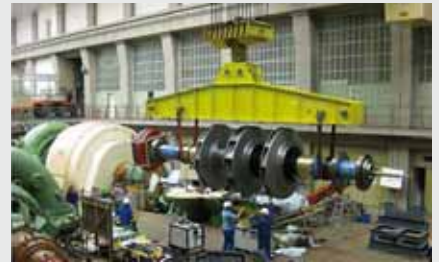
Lifting the refurbished pump rotor into place
