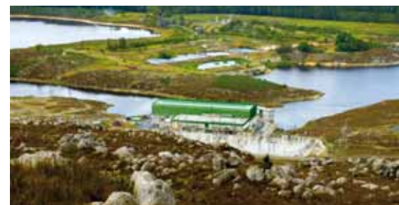
Palmiet pumped storage power plant
