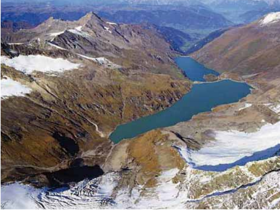
Mooserboden and Wasserfallboden reservoirs
