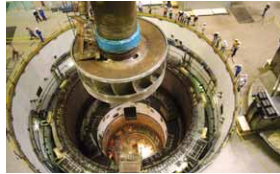
Lowering into turbine pit at site
