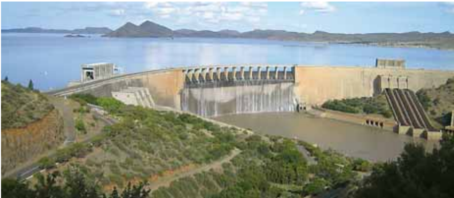
Gariep Dam and power plant
