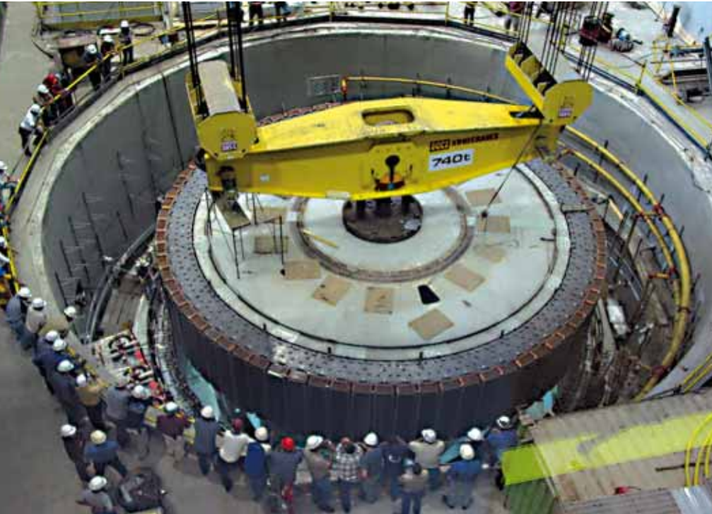
Lifting of a large rotor into pit weighing 630 tons
