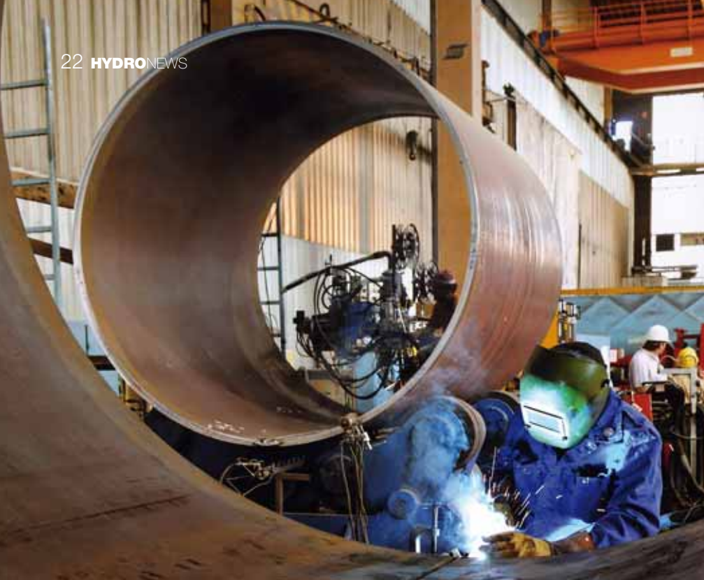
Shop fabrication of pipes
