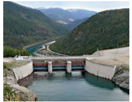
View of Mica Generating Station spillway
