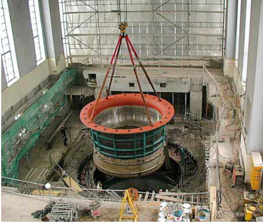
Installation of the discharge ring of the new Kaplan unit
