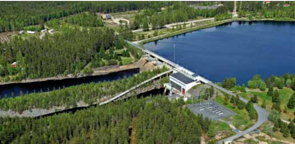
Pahkakoski power station
