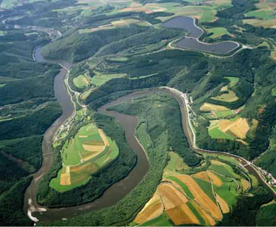
Aerial view of pumped storage power station, Vianden
