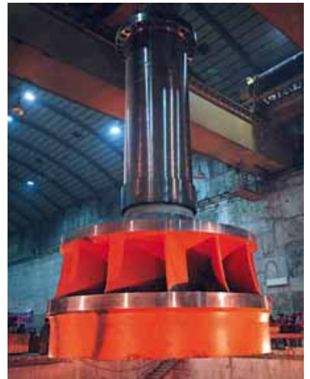
Lifting of runner & shaft weighing 203 tons
