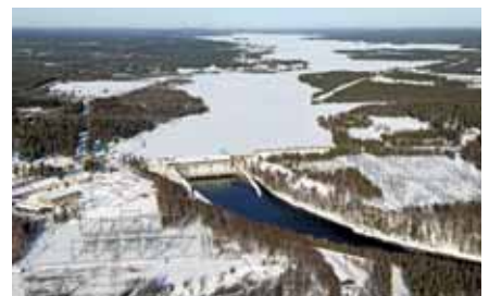
Petäjäsoski power station in wintertime
