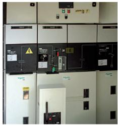
The electrical equipment setup is completed by step-up transformers, high-voltage switchgear, and station service equipment. At the Chievo dam all these systems have been placed in two operation buildings located in close vicinity to the module. The power and control cables of the turbine generator units are run inside of the module gallery and are collectively routed to the landside generator switchgear using a flexible cable chain, cable trays and conduits.
