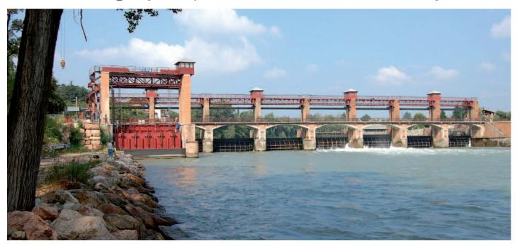
In Verona's district of Chievo a dam and adjacent ship lock were built in the 19th century on the Adige River to establish the Camuzzoni canal. The abandoned ship lock downstream of the Chievo dam owned by Consorzio Canale Camuzzoni was modified to harvest the unused hydropower potential of the abandoned lock without compromising its flood discharge capabilities.
