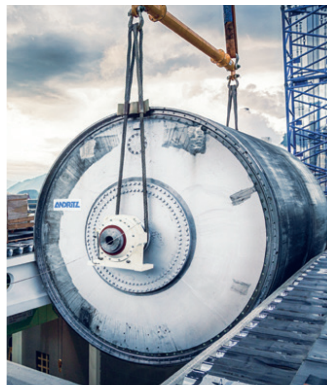
ANDRITZ delivers PrimeDry Steel Yankees with diameters of up to 26 ft.
