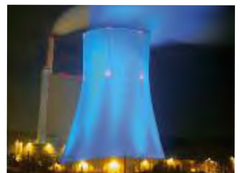
1 x 910 MVA, Bexbach, Germany
